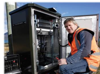
Fig. 15. Securing maintenance data transmission for transportation structures in the nation.
